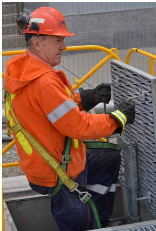
Mick Murray demonstrates the Safe Entry/Exit System's three-point contact.
