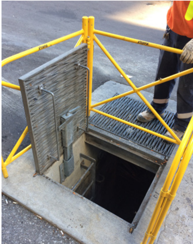
The Safe Entry/Exit System retrofitted to an old lid.
